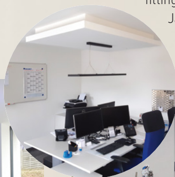
The high-quality equipment includes cooling acoustic ceilings
