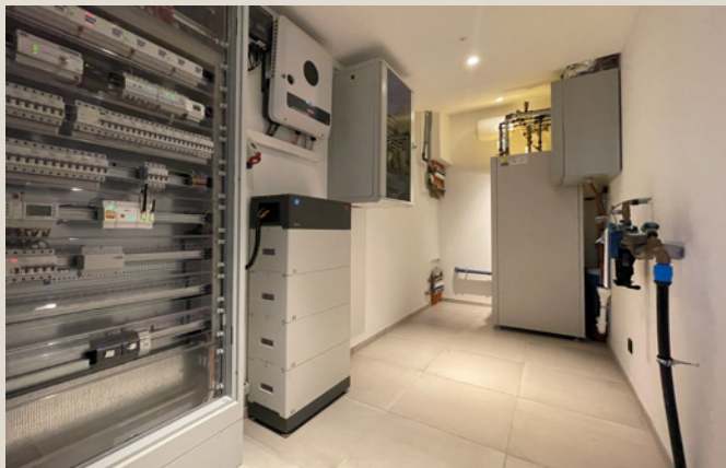
Technology that inspires. Heat pump, storage tank, inverter and two VarioManifold 5.0
