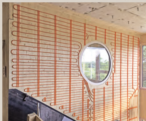
Installing the EasyFlexWall
