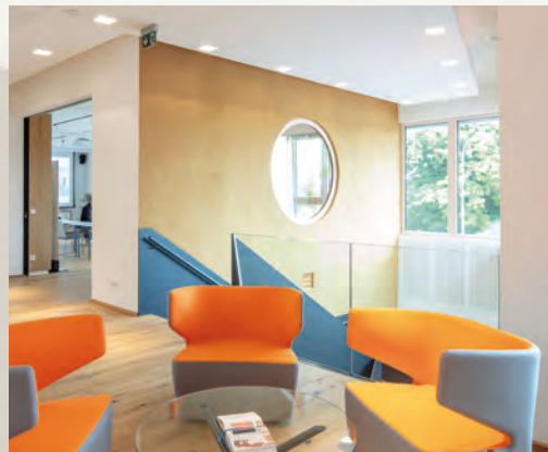
Finished EasyFlexWall with clay plaster
