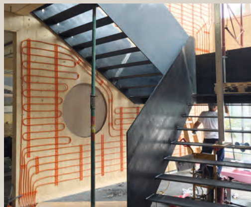
Machine-processed clay plaster also...
