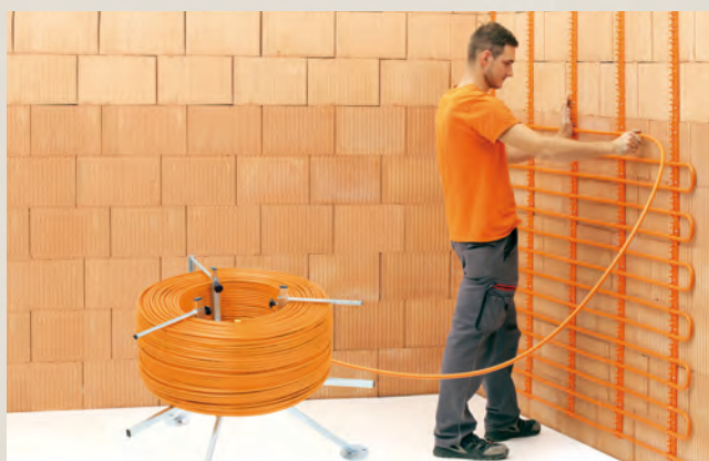
Installing an EasyFlexWall is simple and well thought-out.
